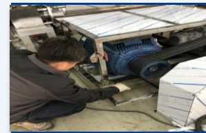
Doing Q/C before installation
